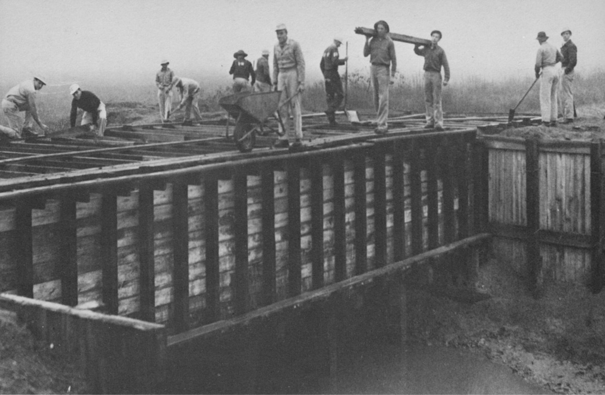
POWs stationed near Alvin worked on the construction of an irrigation canal for nearby rice farmers. U.S. Army Photograph.
